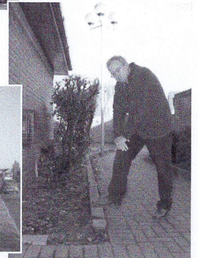
Above: Robin noticed this broken and dangerous path edge at Emperor's Gate and has arranged for it to be repaired
